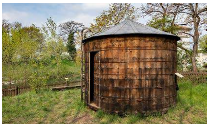
Installation, On Fire-Vulnerable Footage , SALTS, Birsfelden
